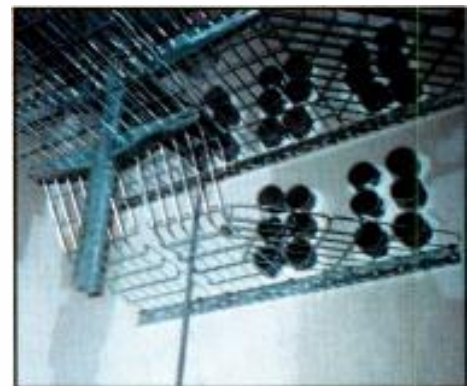
Cable tray assemblies used in the CBS facility. Note the through-wall ports.
